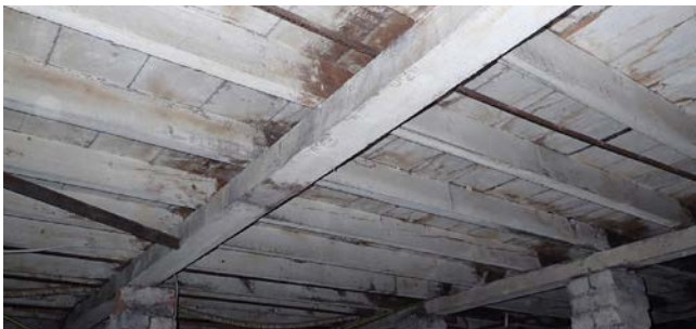
Fig 5. Before the installation.
