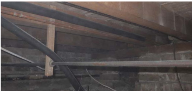
Fig 8. Before the installation.
