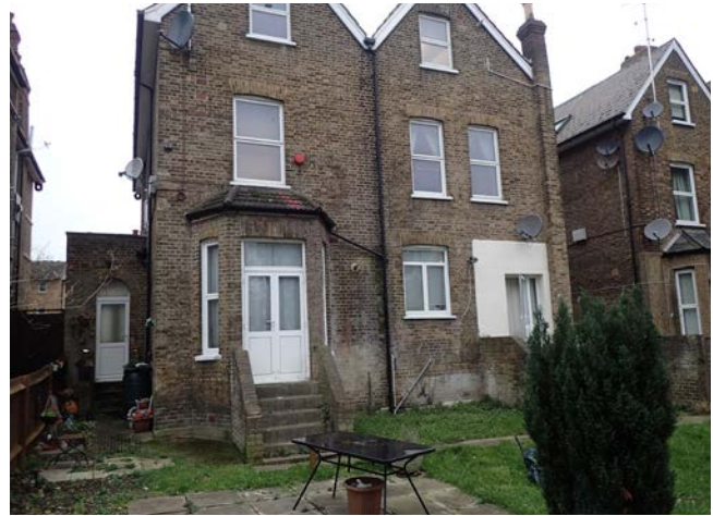
Fig 7. A ground floor flat in converted house.
