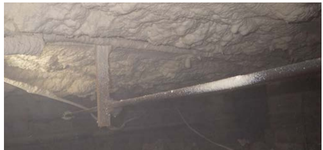
Fig 9. After the installation, showing the insulation now applied.
