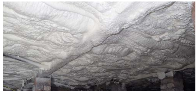
Fig 6. After the installation, showing the insulation now applied.
